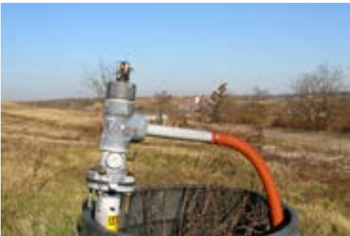
Methane capture at Fresh Kills Landfill
