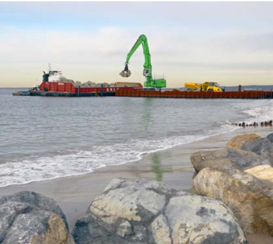
Construction of t-groins at Sea Gate in Brooklyn
