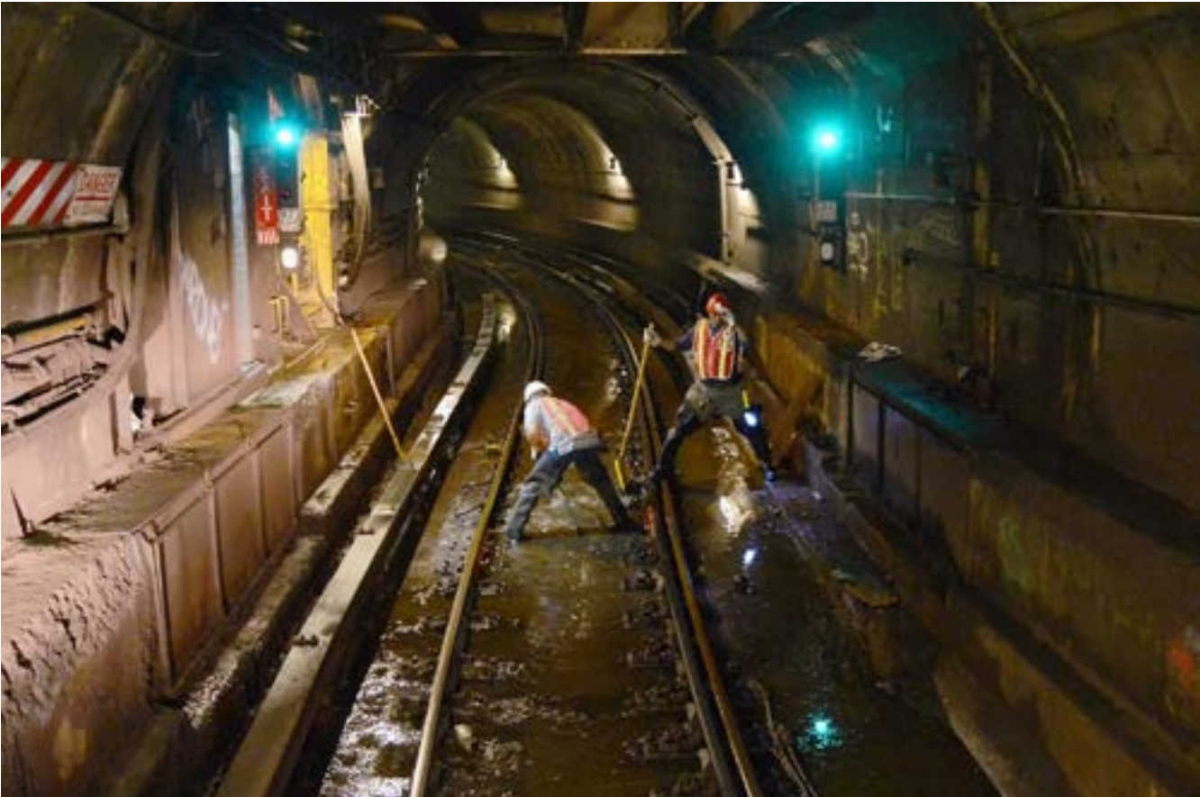
MTA workers clear a clogged drain near the Cortlandt Street subway station to prevent flooding during a heavy rain event
